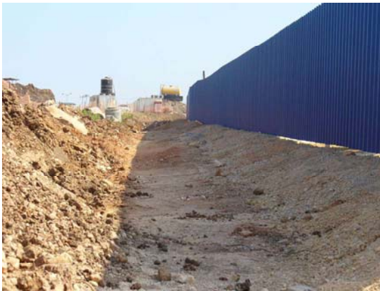
Figure 12: Storm water run-off prevention during construction
