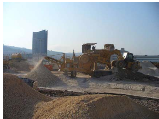
Figure 14: Rock waste crushed on site and recycled
