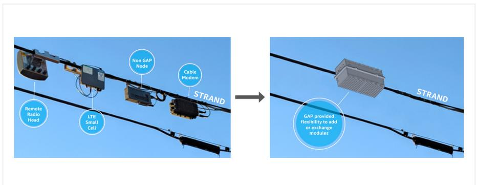
Figure 3. GAP Consolidates Access Technologies
