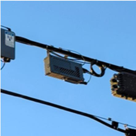
**Figure 1.** Hybrid Fiber-Coaxial (HFC) Node Hangs on Cable Strand
