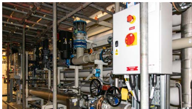
Nanofiltration water system.
