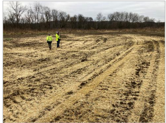
Spot checking grade of middle wetland pool
