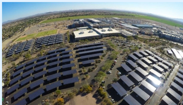
The 7.7-megawatt solar carpark at Intel’s Ocotillo, Arizona campus is made up of 30,000 solar modules covering 3,200 parking spaces. The system was the second largest in the country at time of installation in 2017, with the largest installation at Intel’s campus in Folsom, California.
