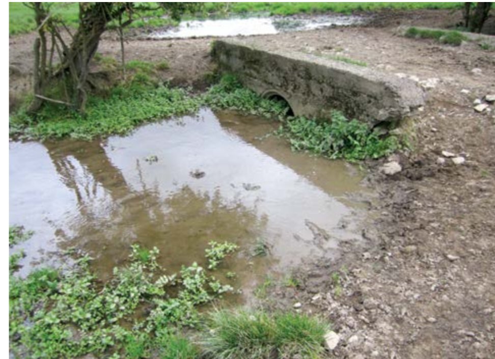
Before and after the removal of sediment, improving flow
