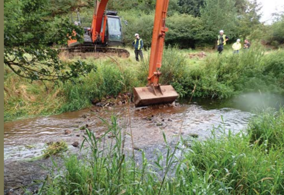
A digger disturbing the sediment at a gravel introduction site
