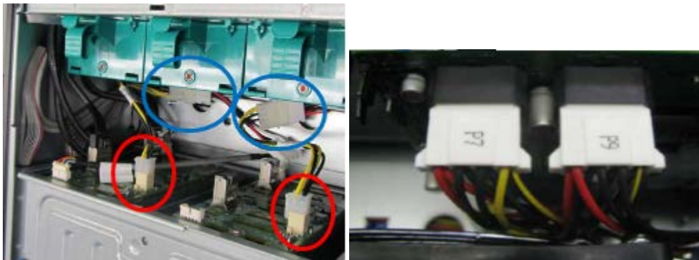
Figure 5. Location examples of the power connectors
