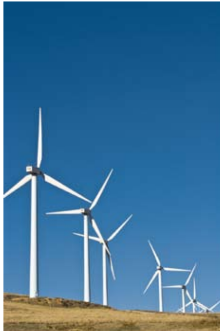
Wind generators are a source of decentralized renewable energy and are also embedded systems in their own right. Sensors and controls are needed to monitor voltage, current and rotation velocity while also reducing dynamic stress on blades, axel, rotors and gearbox.
